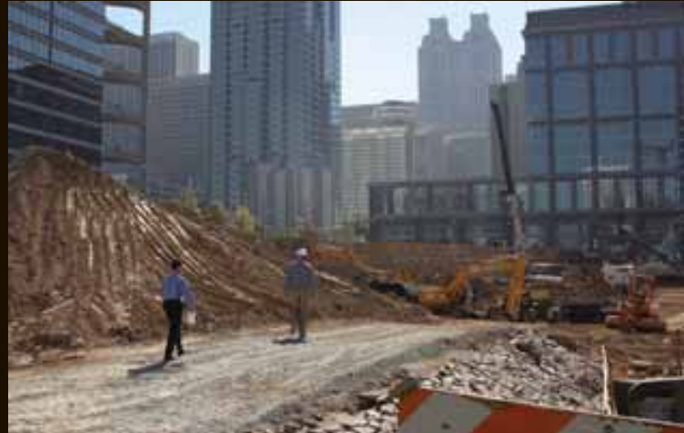
TWELVE Centennial Park broke ground in fall 2005 near downtown Atlanta.
